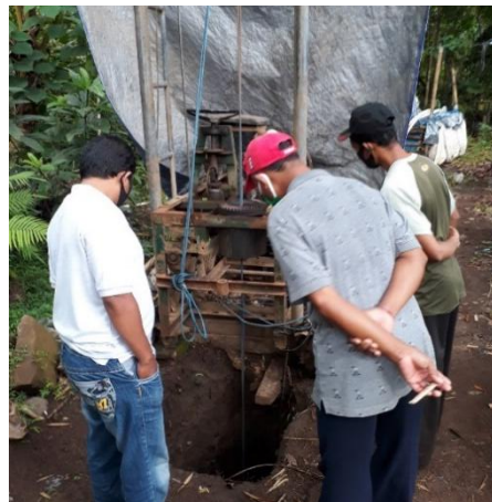
Figure 2. Drilling for Water Sources at Pondok Pesantren At Taqwiin
